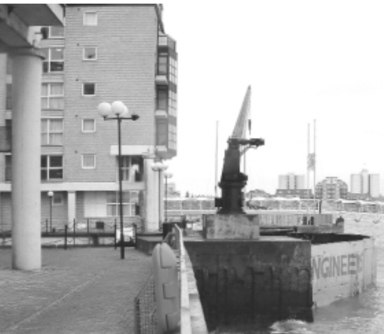
ABOVE: THE CAISSON AT THE ENTRANCE TO THE OLD NELSON DRY DOCK, FROM THE FORMER DANZIG WHARF 2004.
